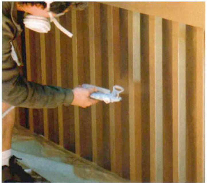
Horizontal, then vertical. Using the painting shield to catch overspray, the author coats the handrail in long, smooth, horizontal strokes (photo left). Then he comes back and coats each side of each baluster in a separate vertical stroke (photo right). After every couple of passes, all surfaces are brushed with a disposable painting pad.
