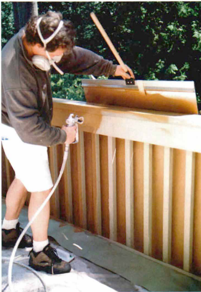
Horizontal, then vertical. Using the painting shield to catch overspray, the author coats the handrail in long, smooth, horizontal strokes (photo left). Then he comes back and coats each side of each baluster in a separate vertical stroke (photo right). After every couple of passes, all surfaces are brushed with a disposable painting pad.
