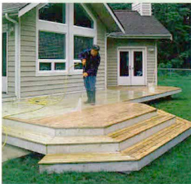
Pressure-washing removes paint and neutralizes stripper.
